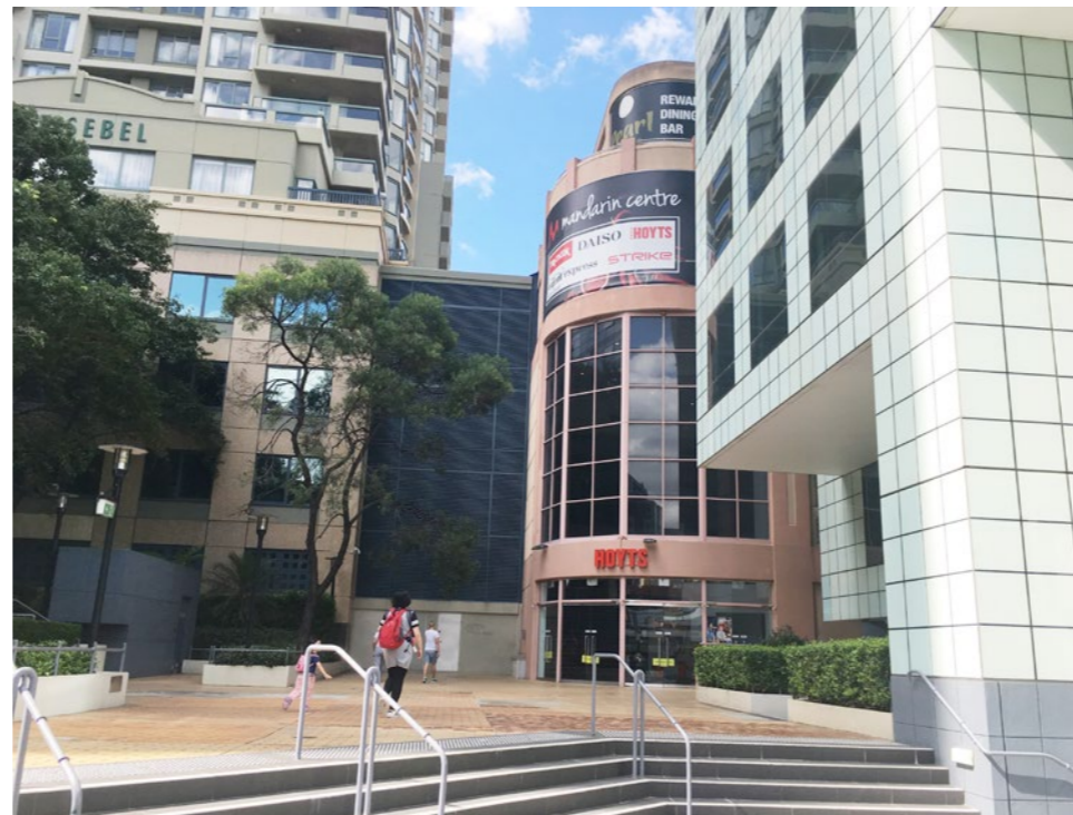
Western corner entrance from Chatswood station approach
