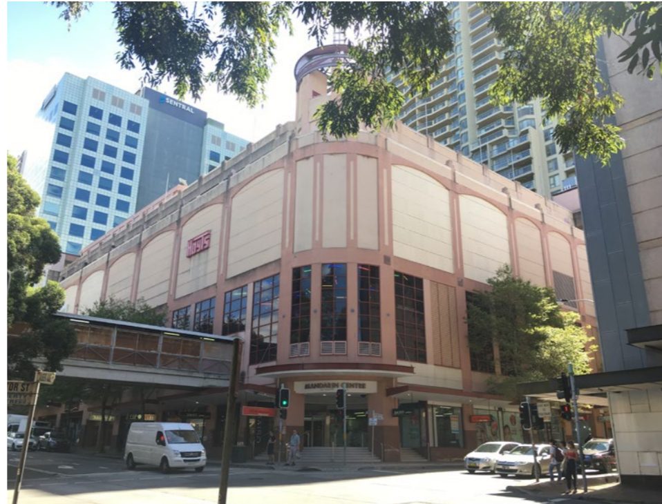
Entrance from the corner of Albert Avenue and Victor Street
